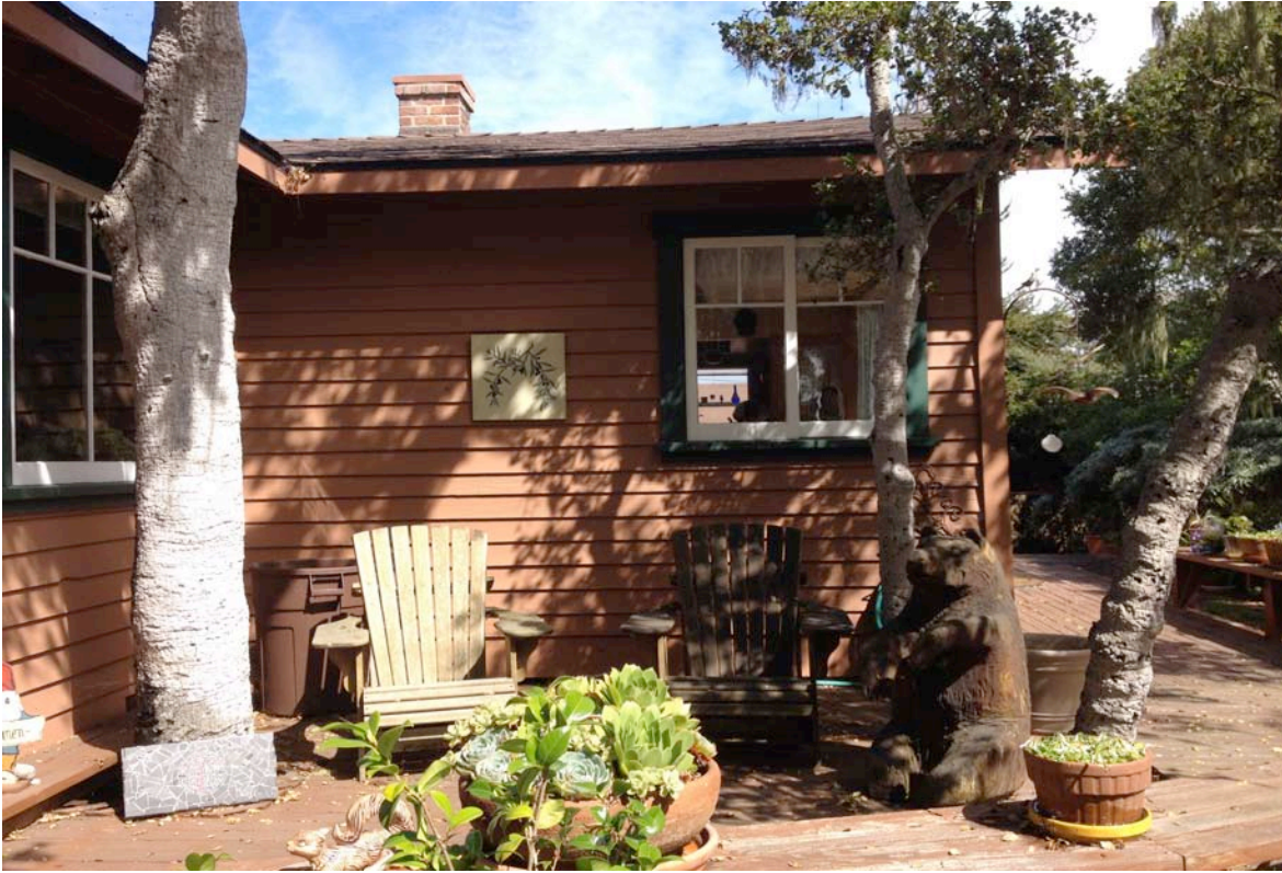
Elevations at Southeast Front Corner
