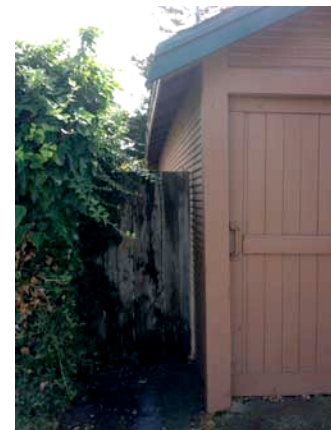
Garage - North Elevation View blocked by fence
